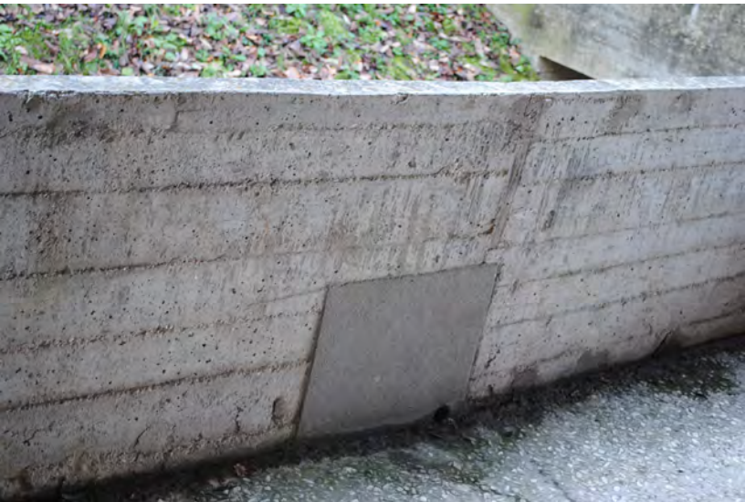
"Colle" residences. Regular repairs patches.
