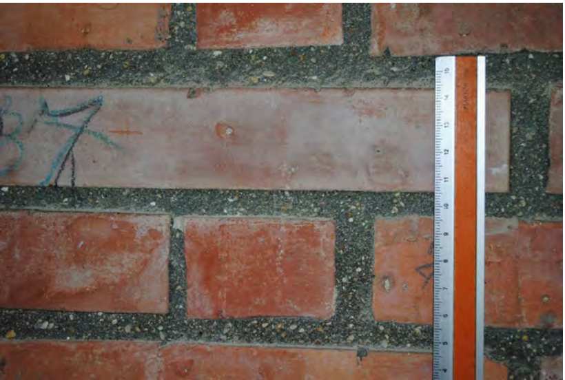
"Colle" (structure). Solid bricks (4 x 11,5 x 24,5 cm) and cement mortar (1 cm).
