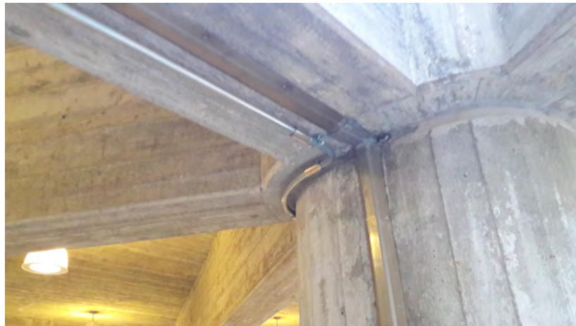
"Tridente" service building. The external surface after the seismic retrofit.
