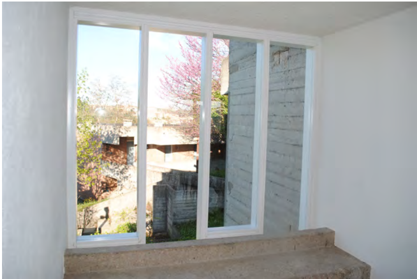
"Colle" service building. The window frames have been replaced with new elements, in wood that has the same dimension of the existing but different opening.
