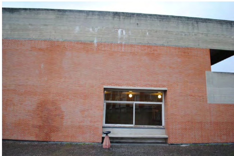
"Tridente" service building. Leaking from the internal drainpipe.
