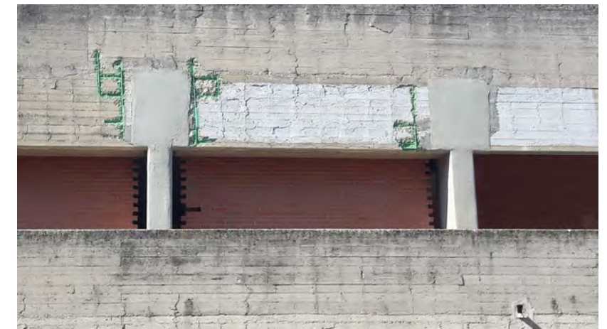
"Tridente" service building. Reinforcement of the structure.
