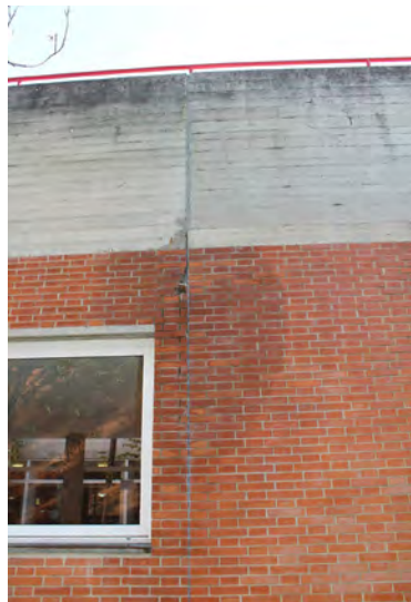
"Tridente" service building. Leaking of water, construction joint.
