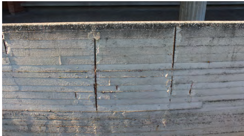
"Tridente". - Corrosion of the rebars and spalling of the concrete.
