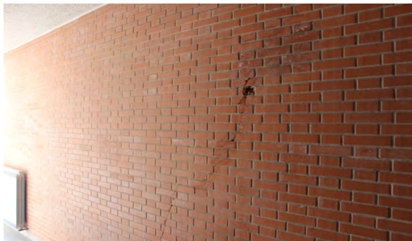
"Aquilone" service building. Cracks.
