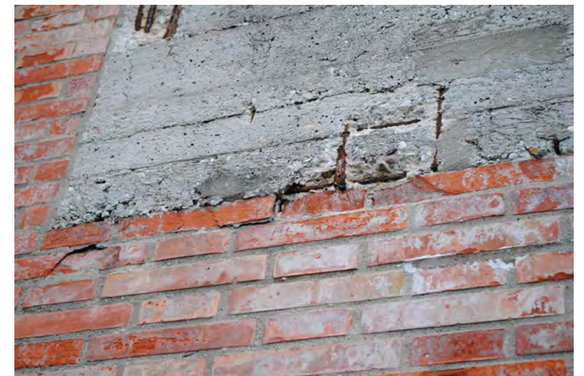
Delamination and efflorescences.
