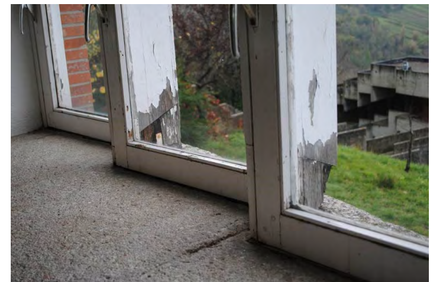
"Colle" service building. Decay of the window frame.
