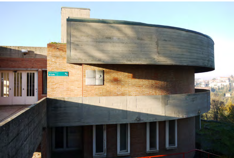
"Colle" service building. The repair patches designed by De Carlo.
