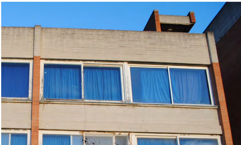
"Aquilone" residences. The trickling of the water causing oxidation and spalling at the center of the concrete slab.
