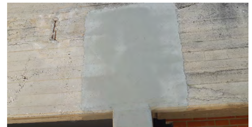
"Tridente" service building. Reinforcements and finishing layer.
