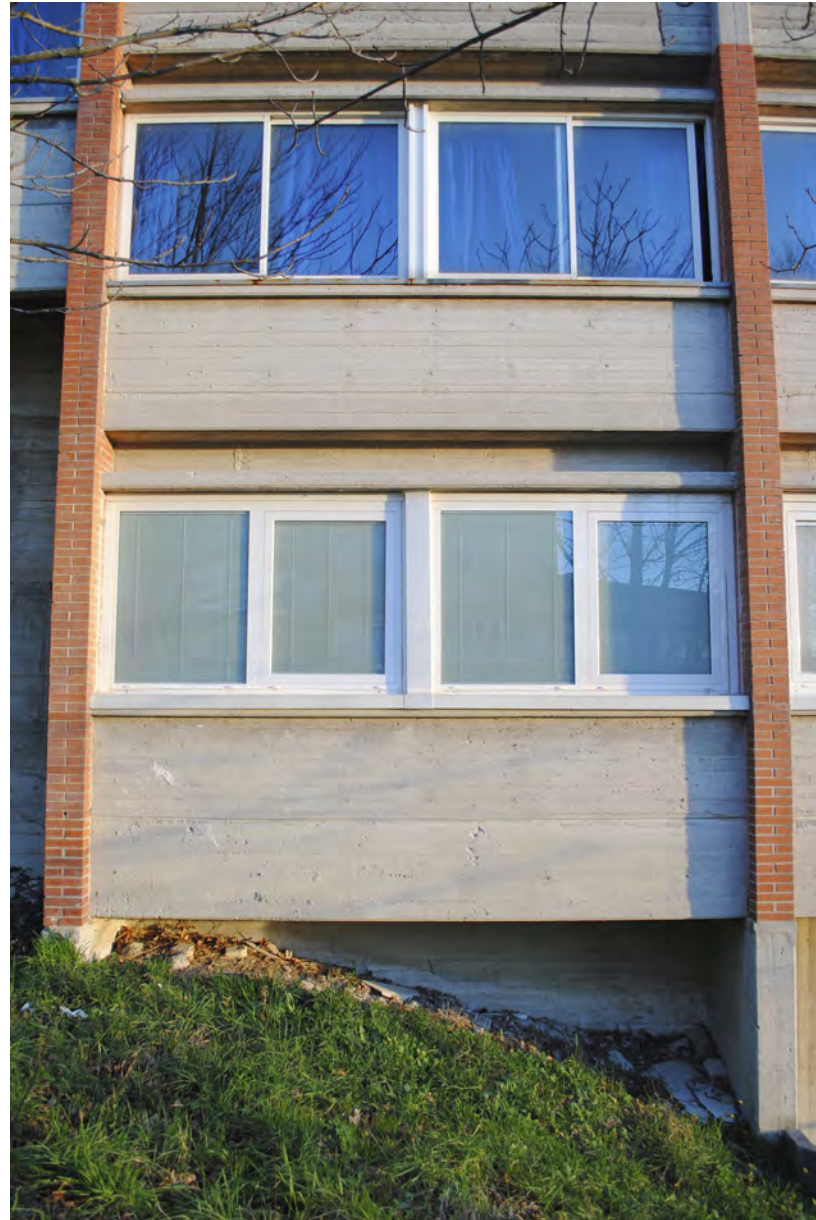
"Tridente". Wooden windows and 2 different types of new windows.
