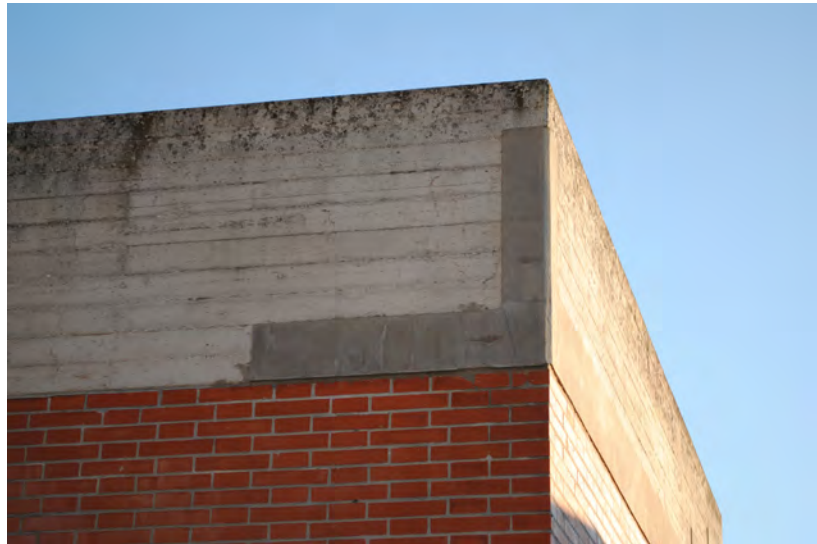
"Serpentine". Regular repairs patches.
