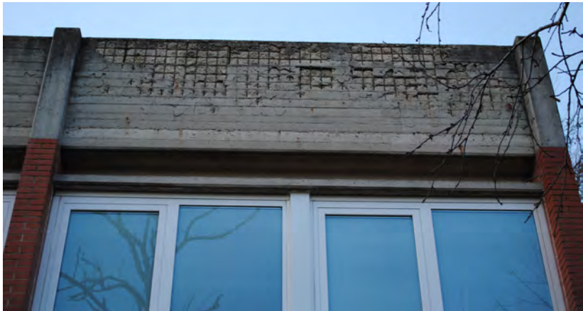
"Nuovi Collegi". Concrete reinforced with a welded steel mesh.
