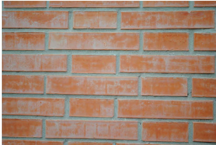
"Nuovi collegi". (structure and cladding, coupled with a concrete structure: hole bricks and cement mortar, 1 cm).
