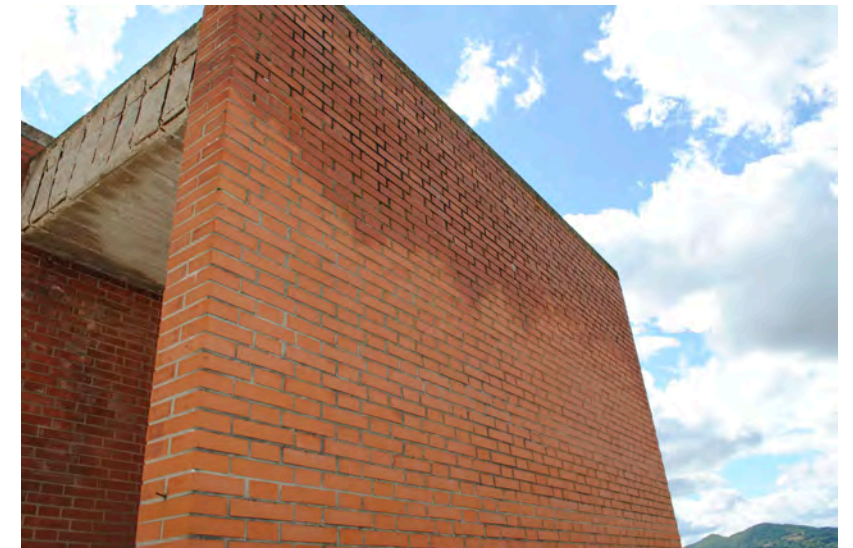
"Aquilone" residences. Stairwell, leaking of water from the roof.
