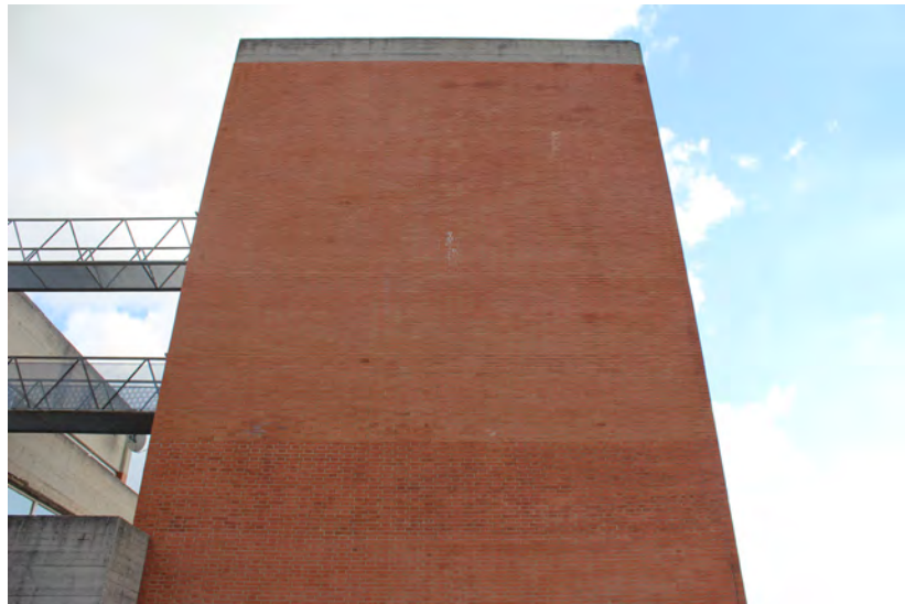
"Vela". Detachment of the cladding from the concrete structure.
